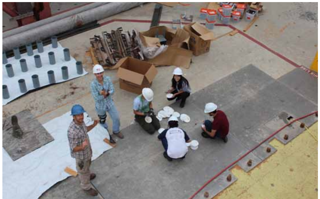
REU students at the NHERI at UC San Diego facility are part of the LHPOST shake table test aiming to develop a seismic design methodology for tall wooden structures. Find details and video on the project: http://nheri.ucsd.edu/projects/current.shtml
