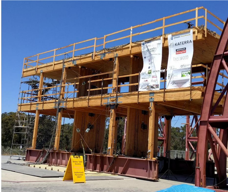
Figure 2. Test structure after the completion of construction and installation of sensors
