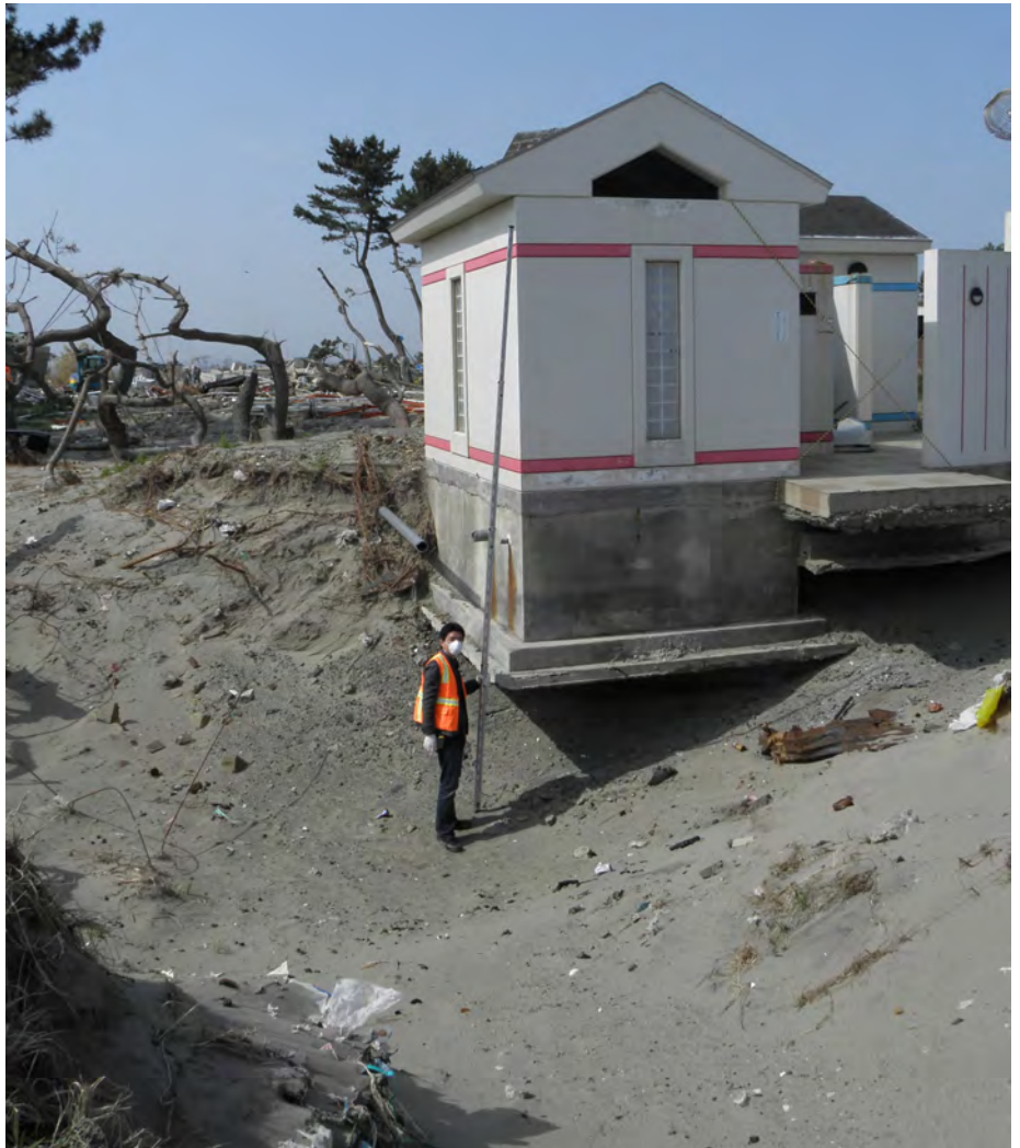
Public bath house near the shoreline of Arahama Beach, Sendai, showing 4m of scour from tsunami (Photo: Lesley Ewing courtesy of American Society of Civil Engineers).
