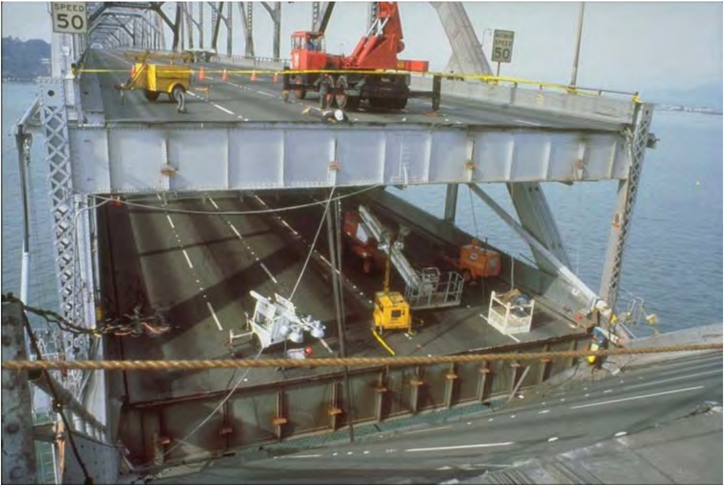
San Francisco Oakland Bay Bridge looking west following the Loma Prieta earthquake. This shows the failed 15-m long section at Pier E-9 (Photo: E. V. Leyendecker, U.S. Geological Survey).
