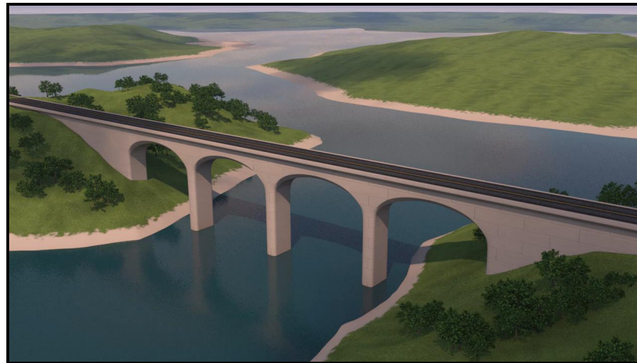
Structural Health Monitoring/Soil-Structure Interaction
