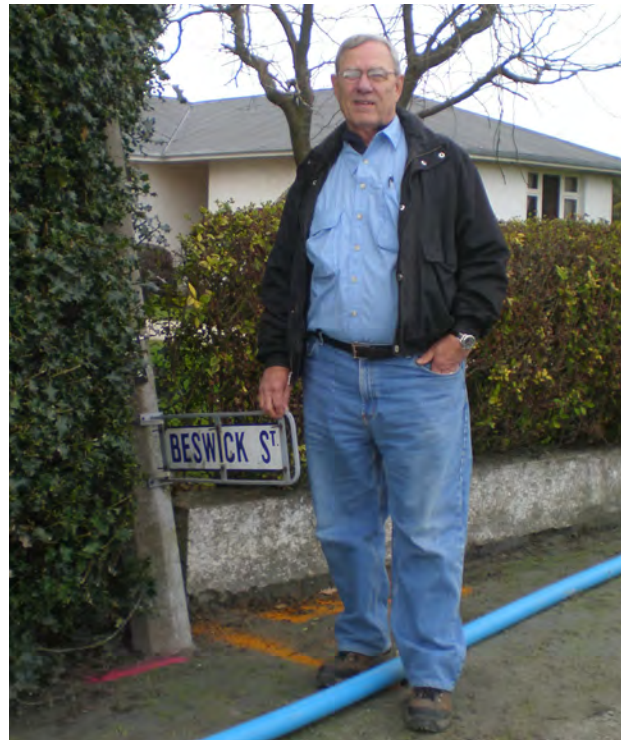
Liquefaction in the Kaiapoi residential area from the 2010 Darfield Earthquake, New Zealand, caused significant damage to underground utilities preventing reoccupancy. This street sign was dropped about six feet straight down (Photo: Bill Holmes).
