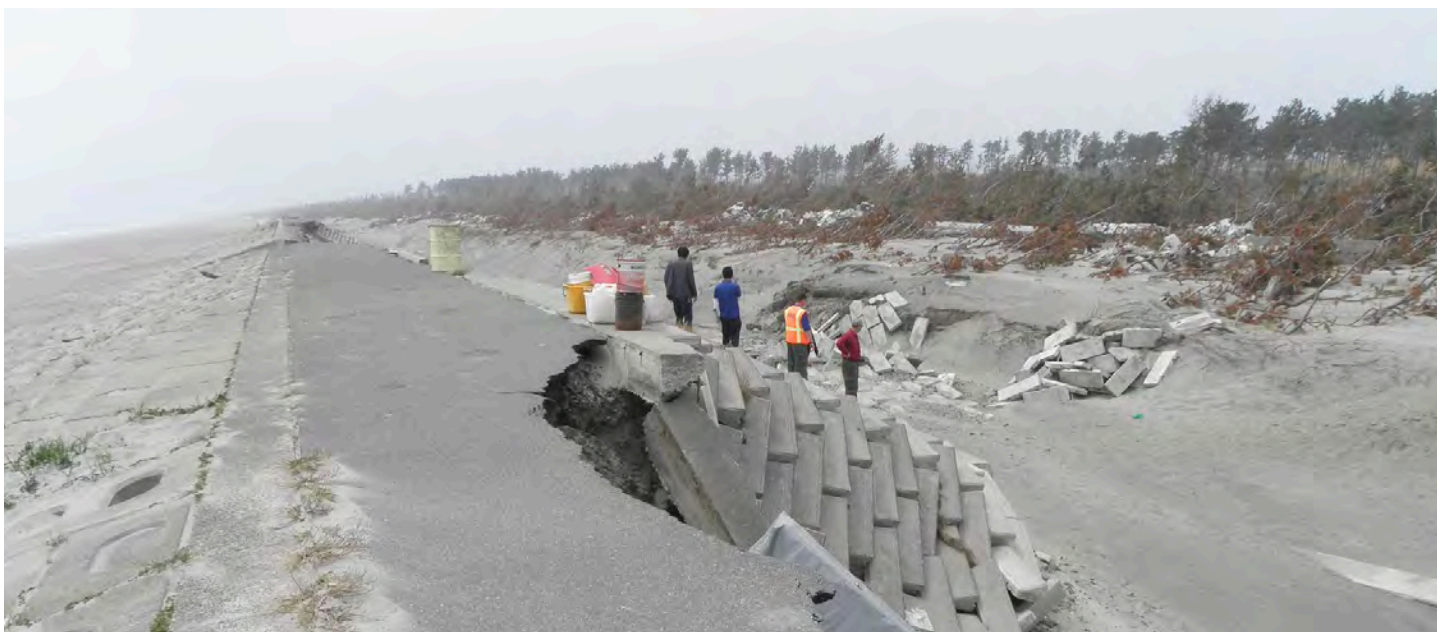
Natori Beach seawall with large amount of scour and damage in the inland side of the seawall. Seaward face of seawall was intact (Photo: Lesley Ewing, courtesy of ASCE).
