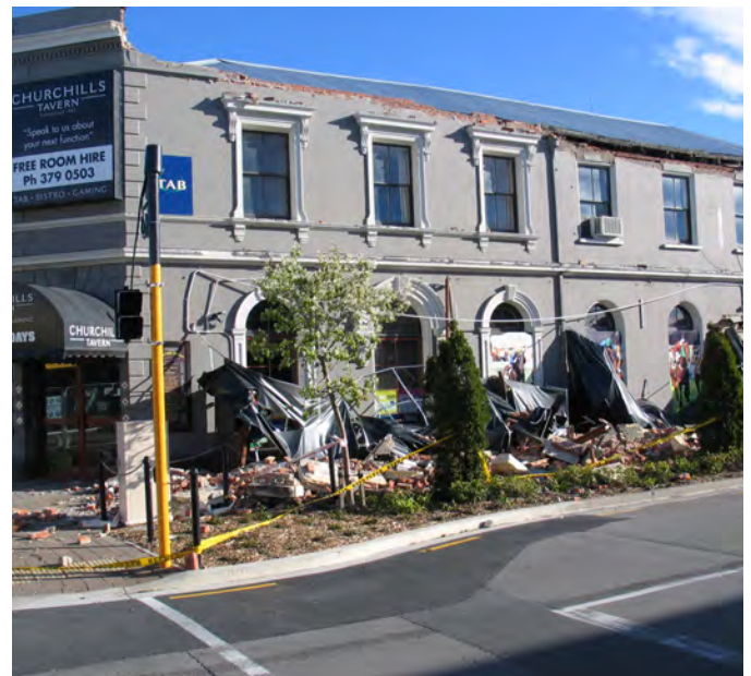
The parapet toppled on to an outdoor seating area. Fortunately, the earthquake occurred at 4:45 am. The most dangerous building type is the older unreinforced masonry bearing wall building, still common in regions of high seismicity (Photo: Bill Holmes).
